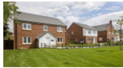
Crest - Lower Road East
