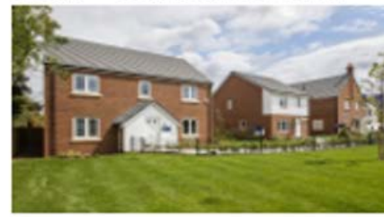
Crest - Lower Road East
